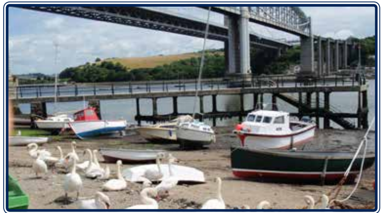
17 Saltash and the Tamar Bridge
