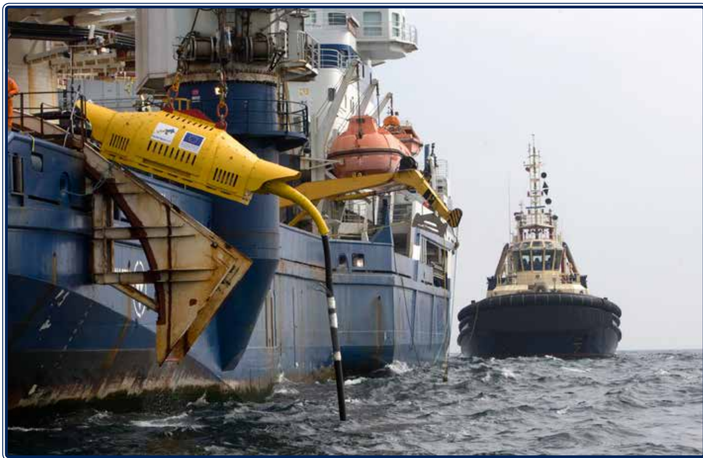
19 Installation of the Wave Hub off Hayle Harbour
