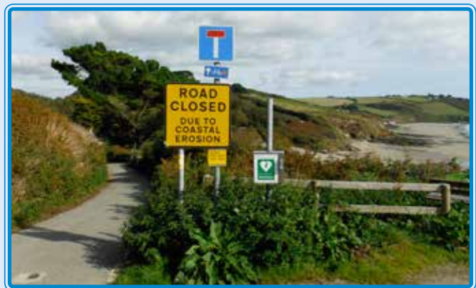
12 Erosion sign, Pendower, Roseland
